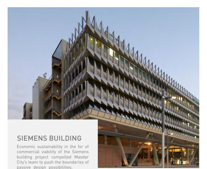
The Siemens Building is compact in form, being practically square on plan. Compact buildings can lead to less façade area which, in the case of Masdar City, reduces heat transfer from the exterior to the interior of the building. This approach to passive design also has cost benefits since less façade area requires less quantities of construction material to complete the building envelope.
